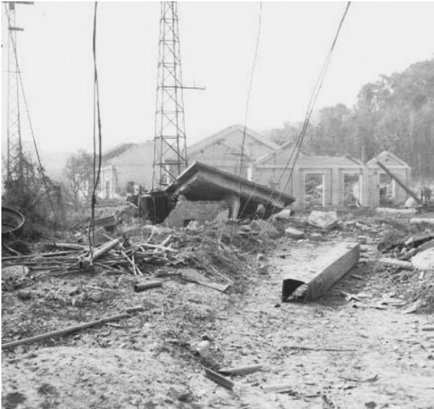
Fig. 3. Electric power room. Picture taken 80 m from epicenter.
