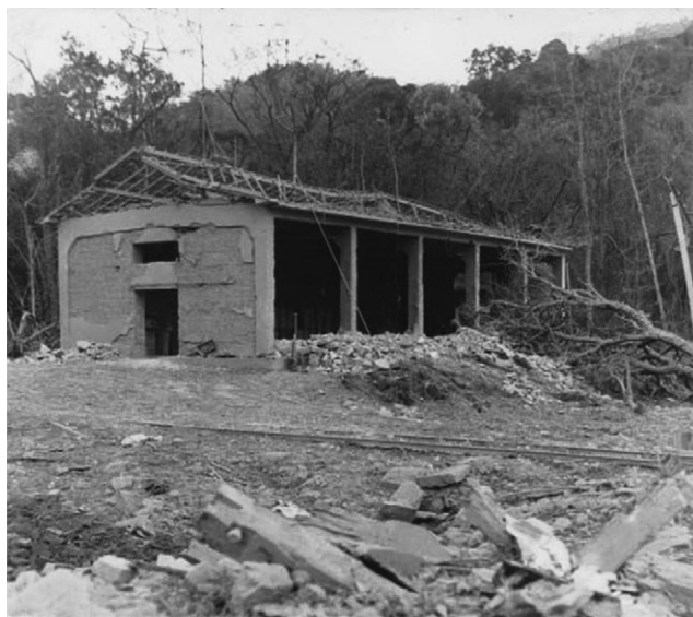
Fig. 1. Single base powder boxes storage depot. Picture taken 50 m from epicenter.
