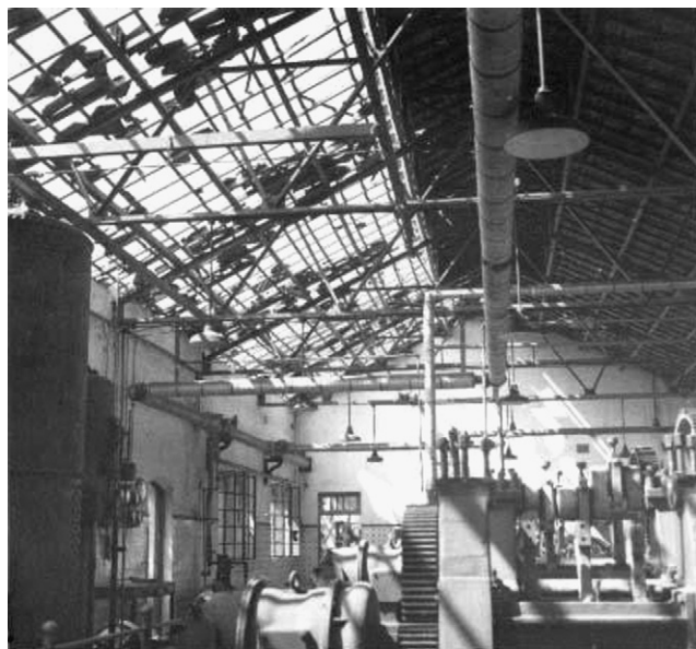
Fig. 12. Boiler room. Picture taken 340 m from epicenter.
