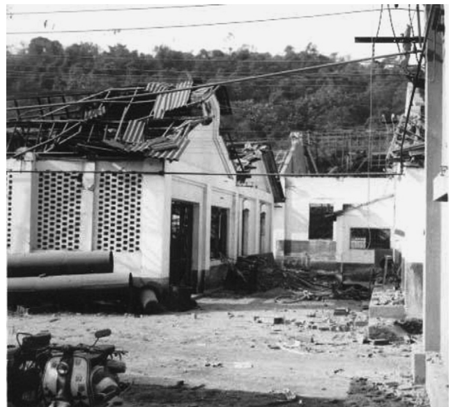
Fig. 6. Machine shop III. Picture taken 170 m from epicenter.
